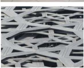
Detail of the dome structure. The columns holding the dome are hidden so the dome really does look as though it is 'floating'
